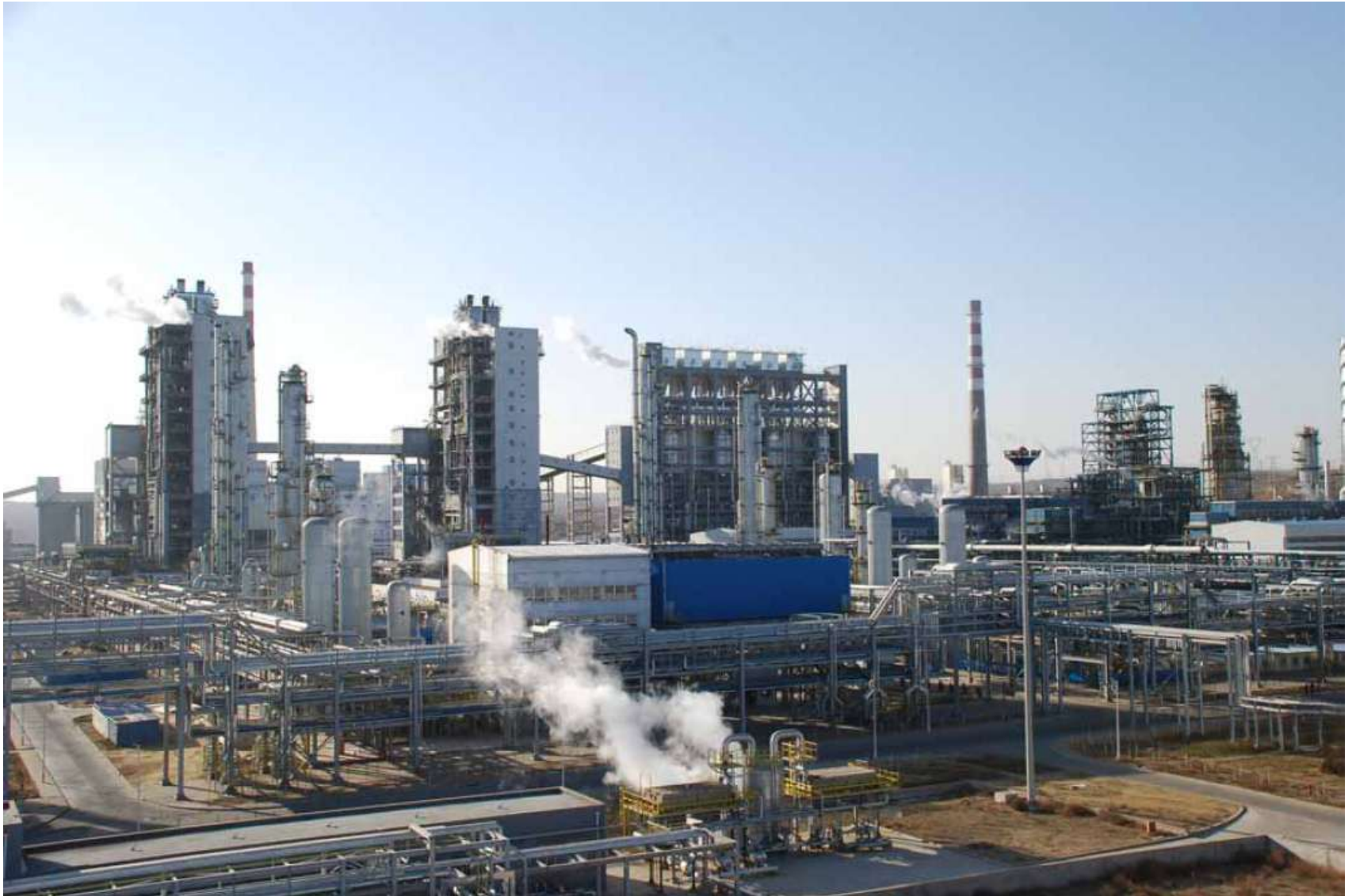
Full View of Coal Liquefaction Plant in Operation
